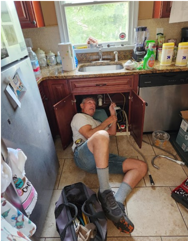
Bob Little fixing the kitchen sink plumbing
